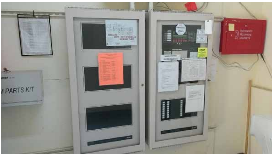
Fire Alarm Control Panel
