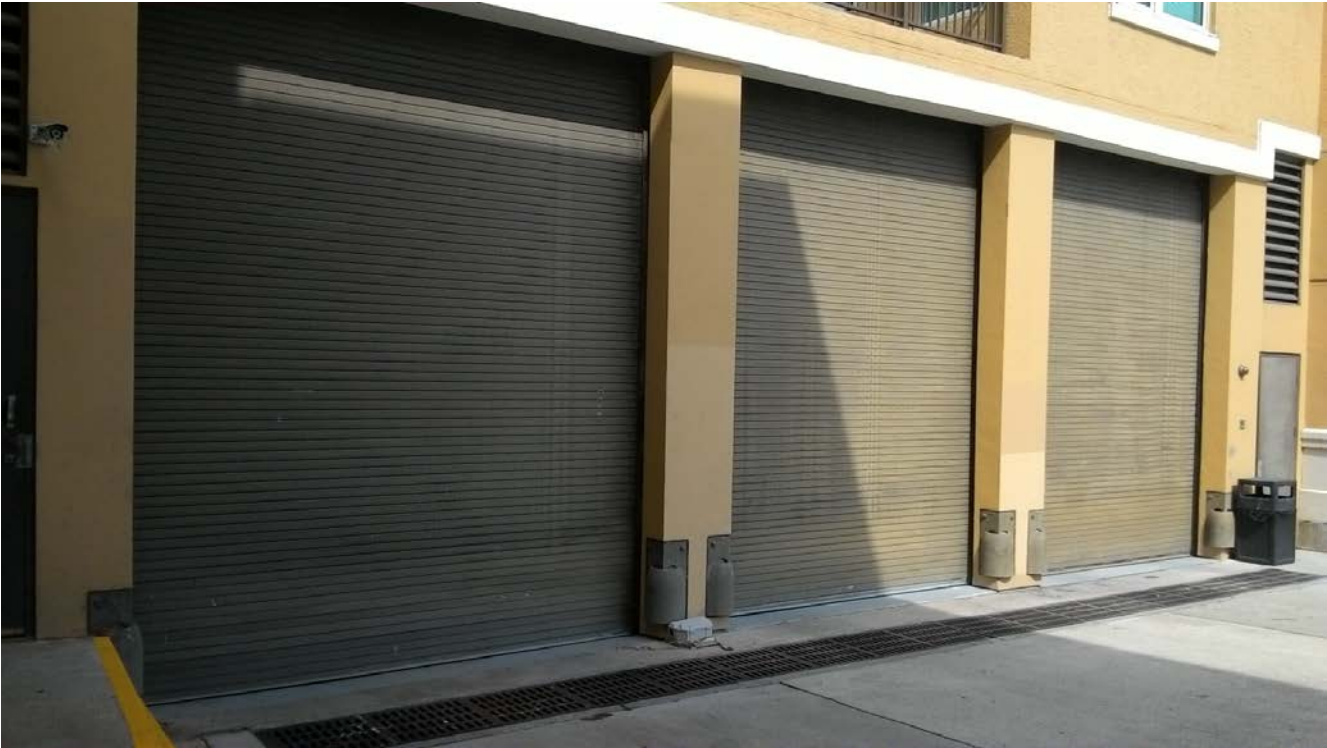
Loading Dock Gates
