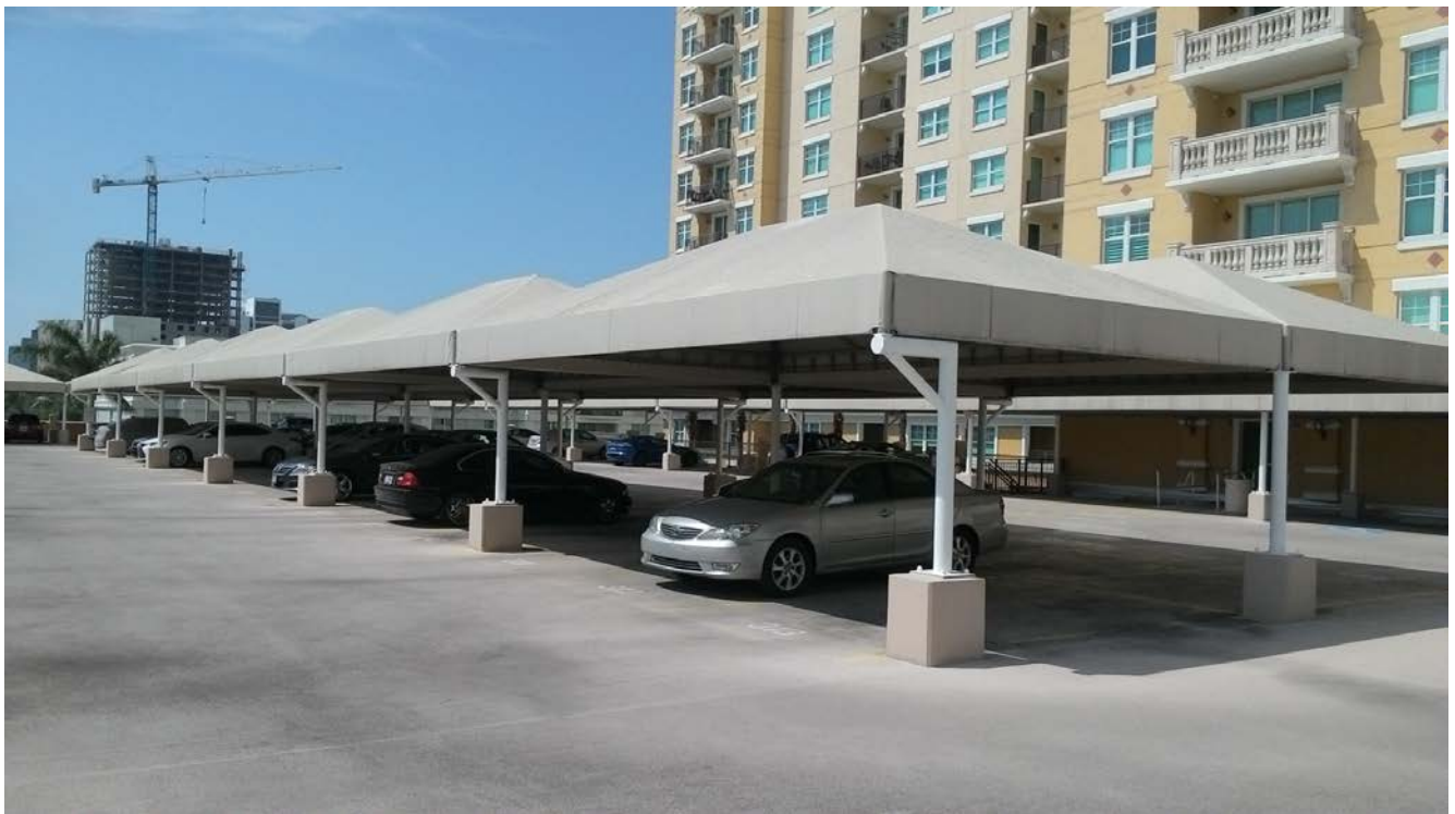
Awnings - Parking Garage
