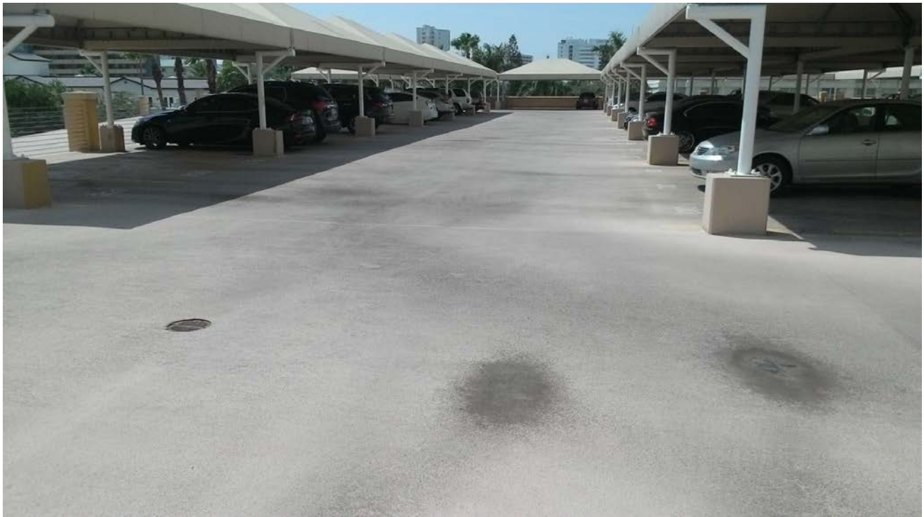
Parking Deck Coating
