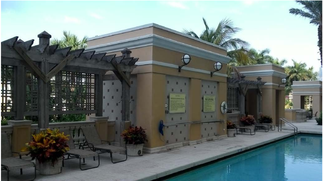
Pool Equipment Bldg
