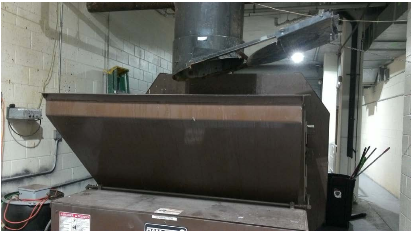
Trash Compactor/Chute
